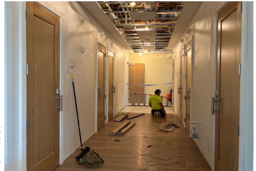
Flooring Under Way at Restroom Corridor
