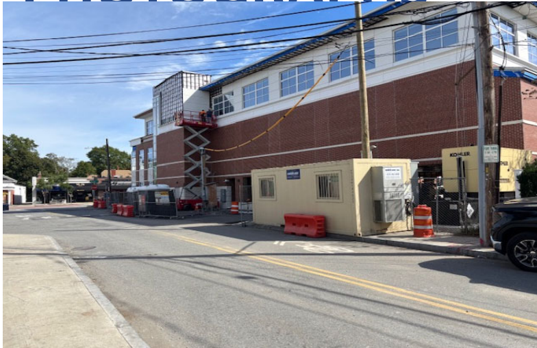
Exterior Panels and Cornice Ongoing
