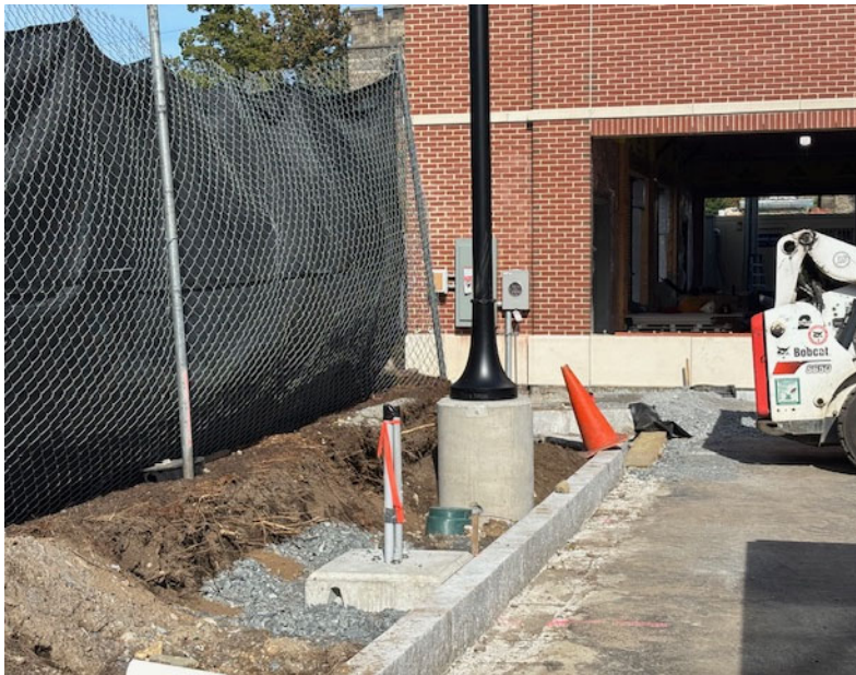
Binder Coat Paving Complete, Lights & EV Charger Install Ongoing
