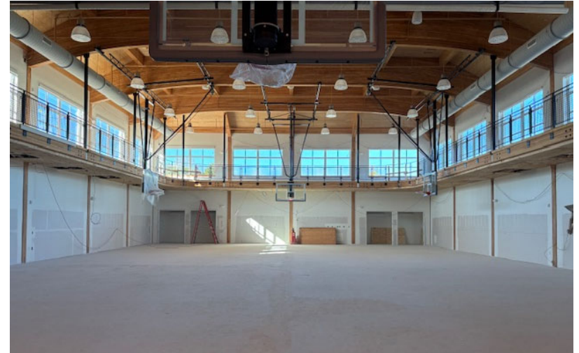
Gym Ceiling Work Complete, Flooring to Begin
