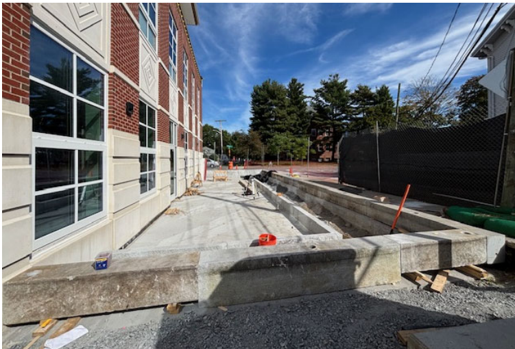
Exterior Patio Curbing Installed
