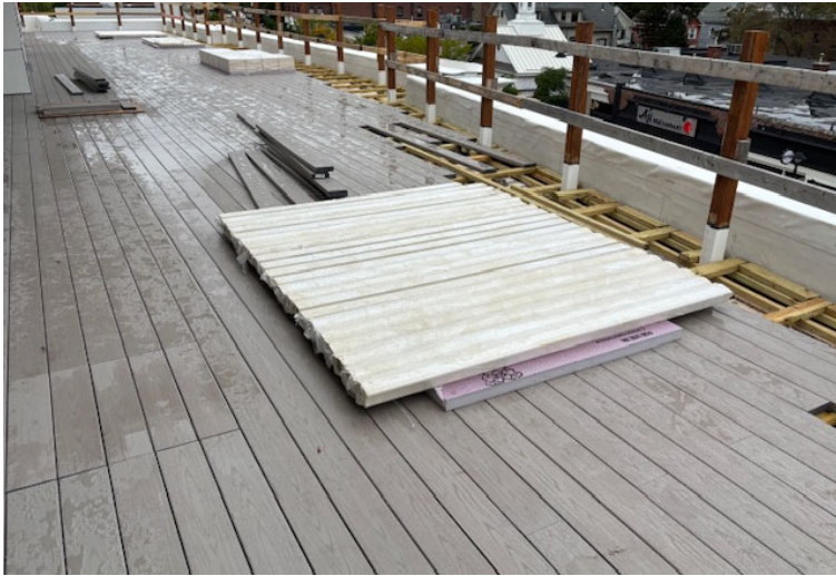
Roof Decking Installed, Railings Ongoing
