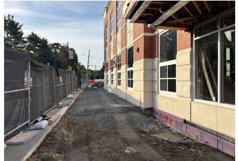
Final grading Ongoing at Front of Building
