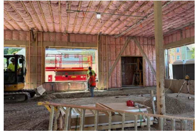
Insulation Installed at Gym over Parking Area
