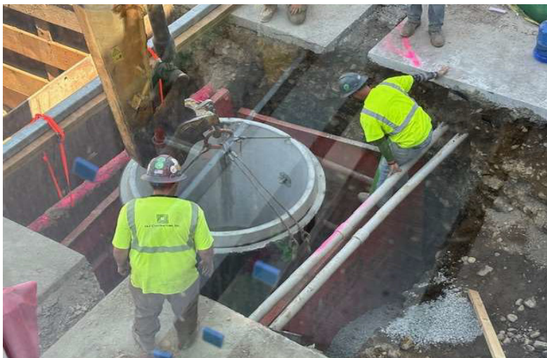
Installation of Sewer Manhole in Highland Ave.
