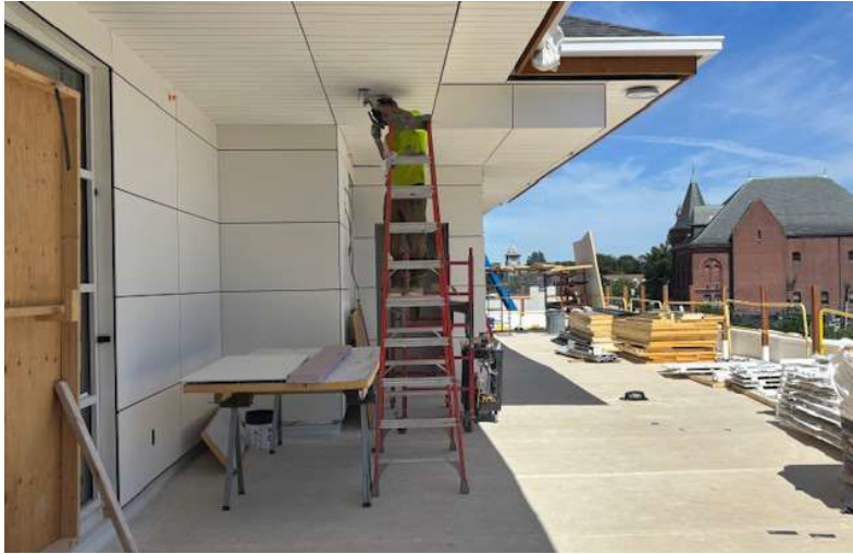
Installing Exterior Soffit Lighting
