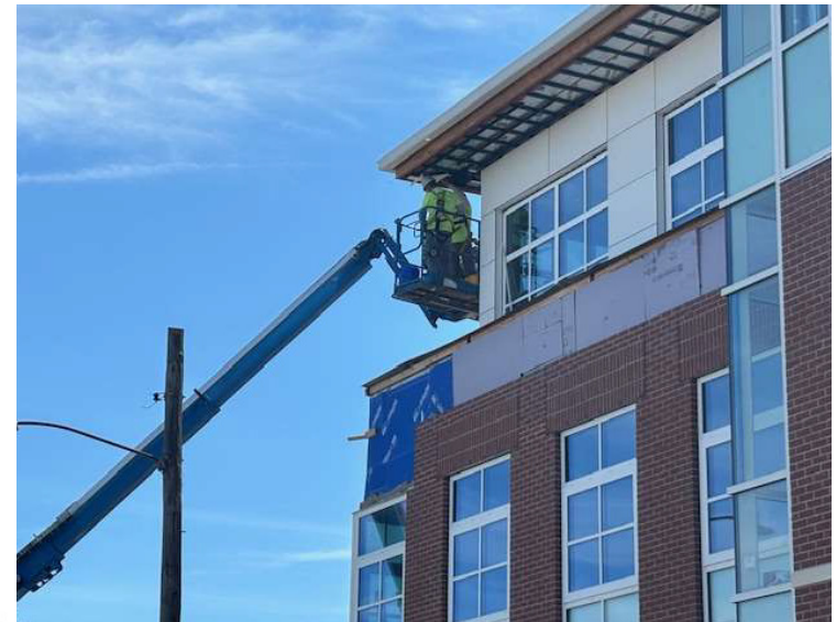
Installation of Exterior Soffit
