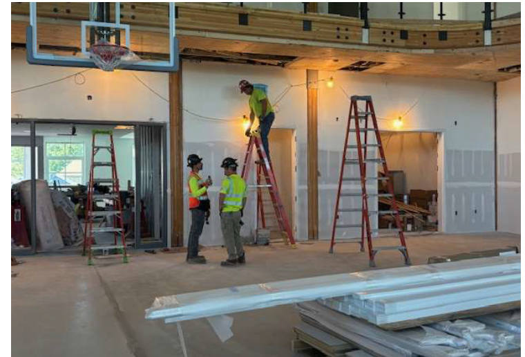
Final Wiring in Gym
