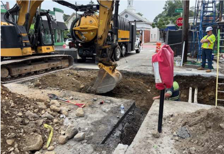
Excavation for Sewer Work in Highland Ave
