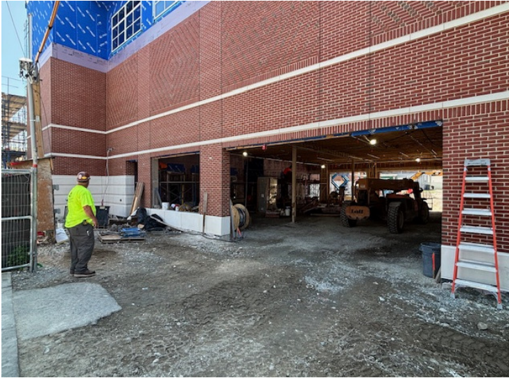
Brick at North Parking Entry nearly complete
