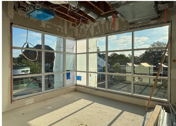
Interior View at Meeting Room
