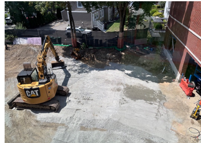
Backfilling complete over Infiltration System
