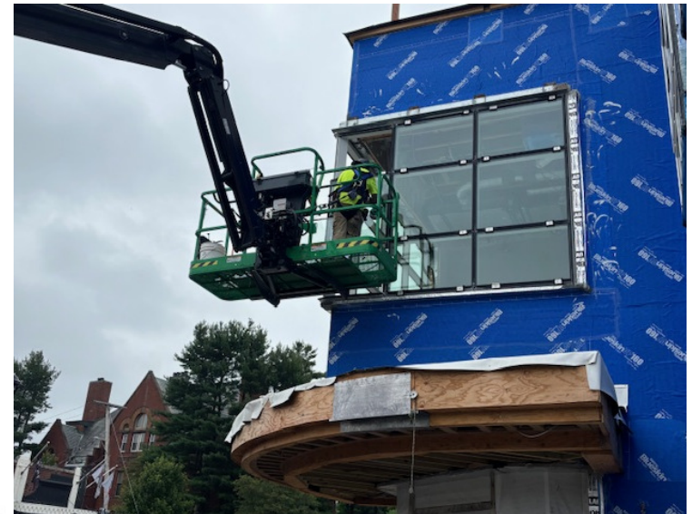
Curtainwall Installation at Meeting Room
