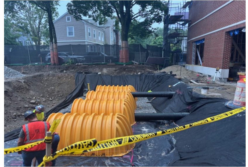
Infiltration System Structures and Piping Installed
