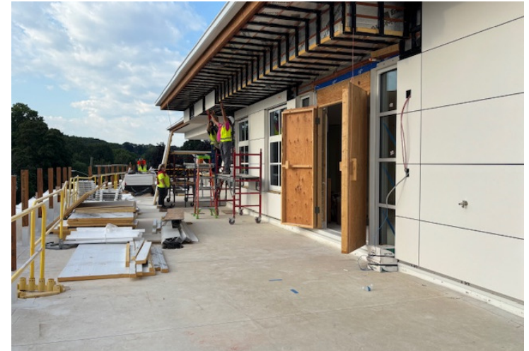
Wall and Ceiling Panels Under Way at Roof Deck
