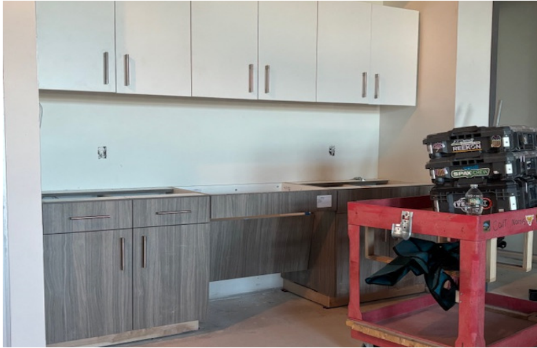
Finish Casework Ongoing
