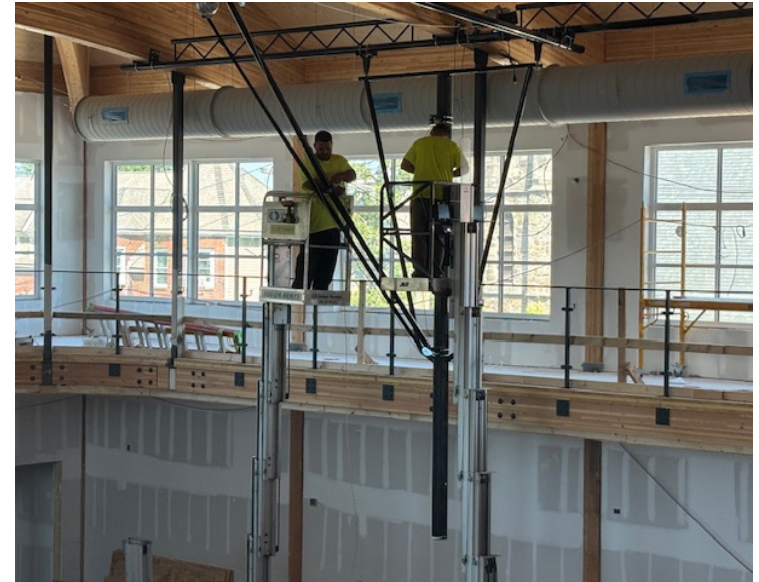
Gym Athletic Equipment Installation
