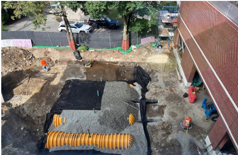
Infiltration System backfill with crushed stone
