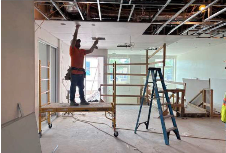
Gypsum board Ceiling Installation on Second Floor
