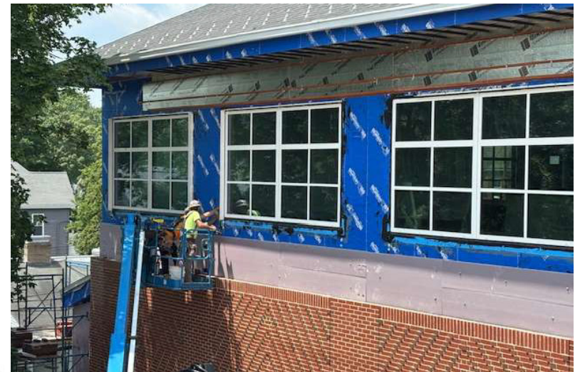
Masonry Complete/Cement Panel Installation on South Gym
