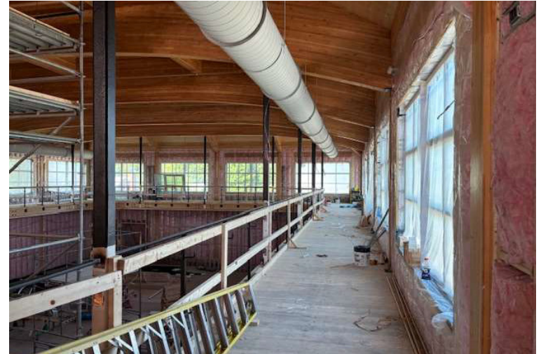
Ductwork Installed in Gym
