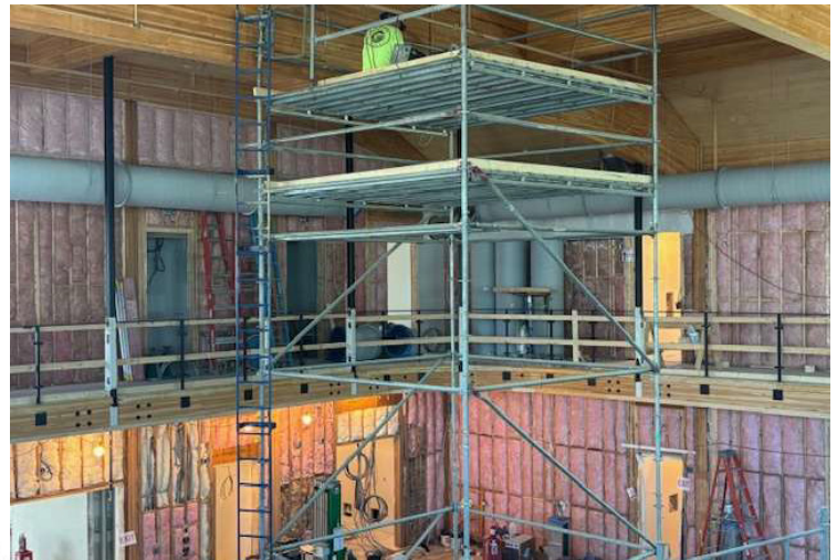
Conduit and Electrical Work at Gym Ceiling
