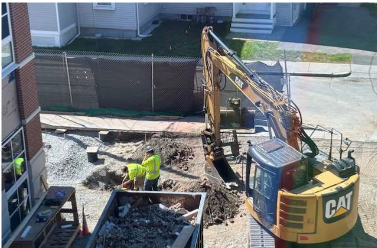
Excavation for Electrical Main
