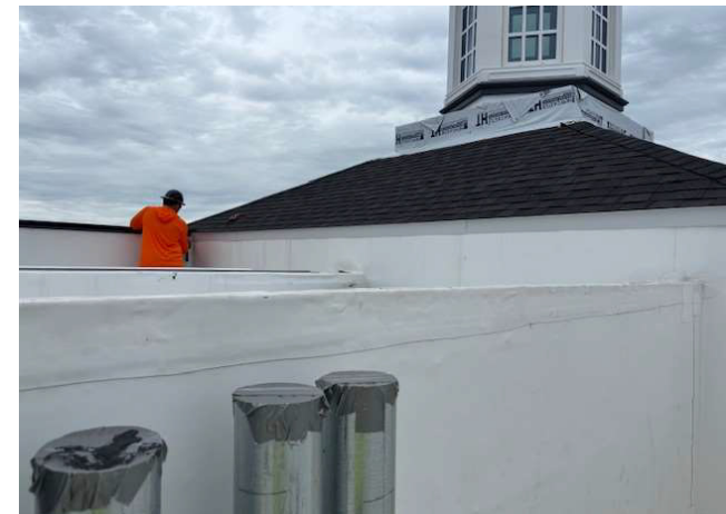
Roofing Trim Work Nearly Complete
