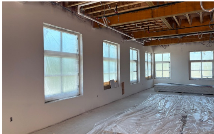
Fitness Room Painting Ongoing
