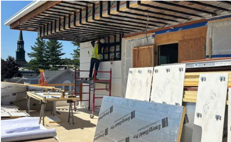
Cement Panel Installation at Roof Deck
