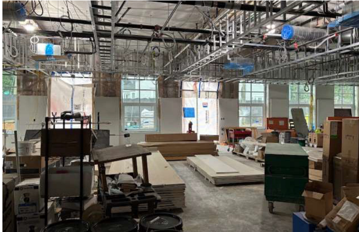
Rough-in at Multi- Purpose Room Complete
