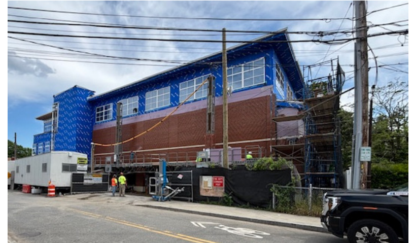
Masonry Complete on Gym North Elevation
