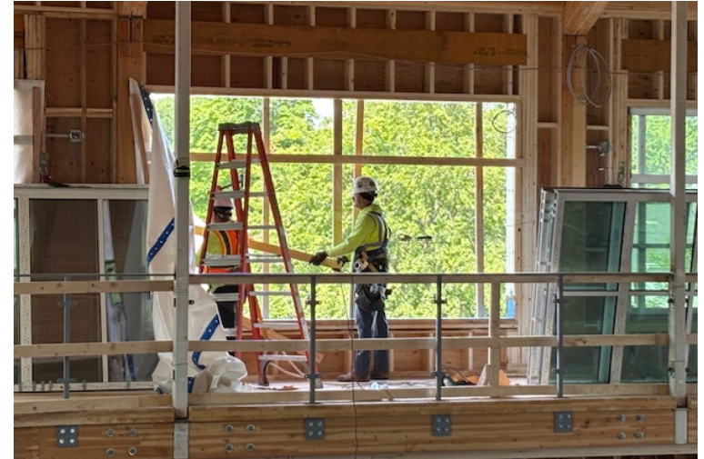
Window Installation at Gym
