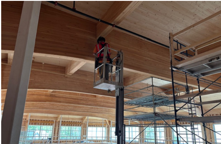
Applying Sealant on Gym Wood Components
