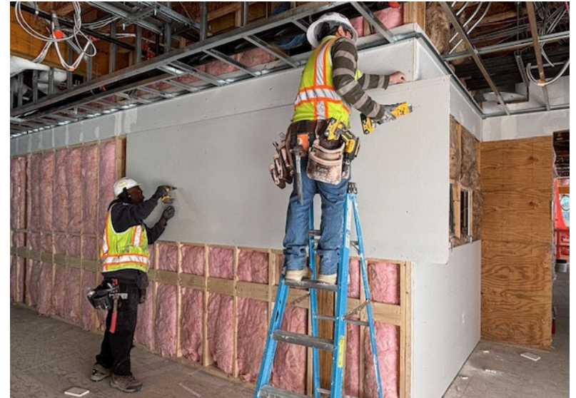
Drywall Installation on Walls
