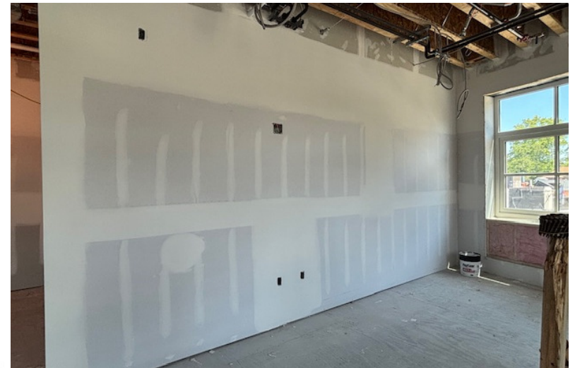
Drywall Taped and Ready for Prime Painting
