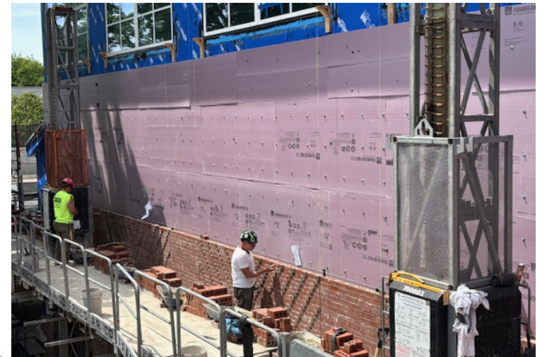
Brick Installation on South Gym Wall
