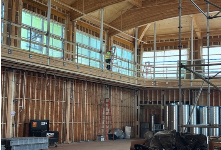
Window Installation in Gym
