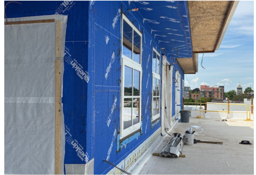
AVB complete on Third Floor at Roof Deck
