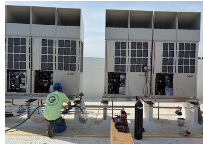
Connecting HVAC Equipment on Roof
