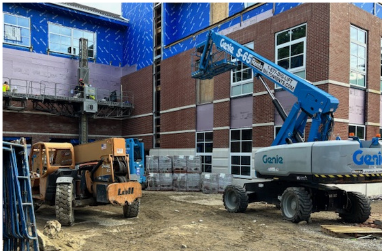
Brick Installation on South Gym Wall
