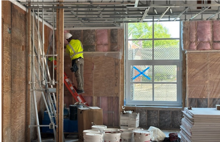
Ceiling Soffit Framing
