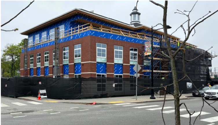
Exterior View from Southeast
