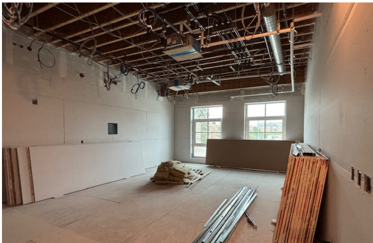
Drywall in Activity Room
