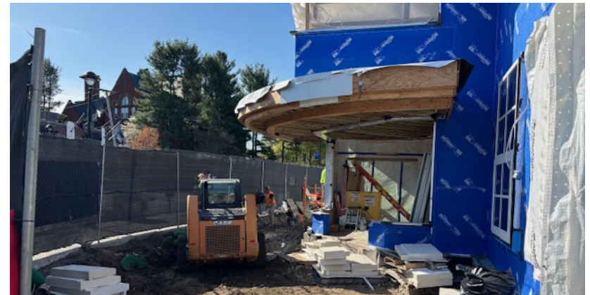
Entry Canopy Roofing Under Way
