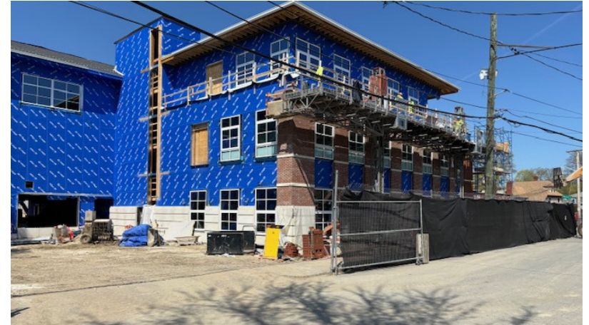
Masonry Installation on South Elevation
