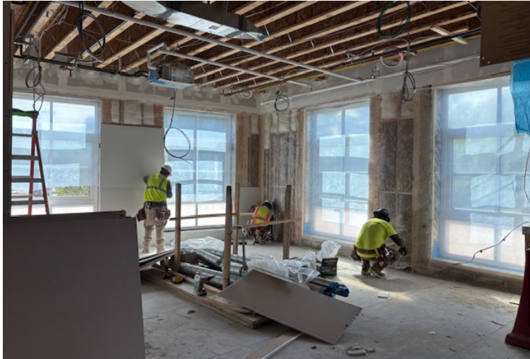
Drywall Installation in Fitness Room
