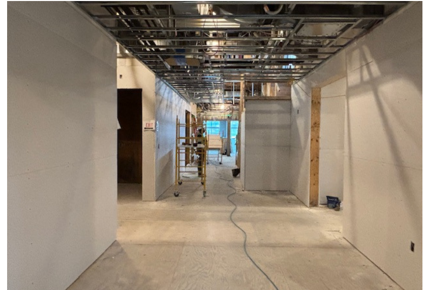
Drywall on Second Floor
