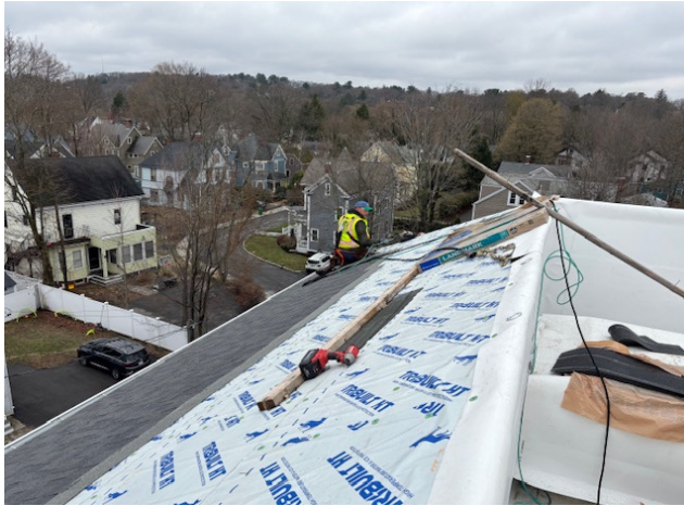
Shingle work on main building
