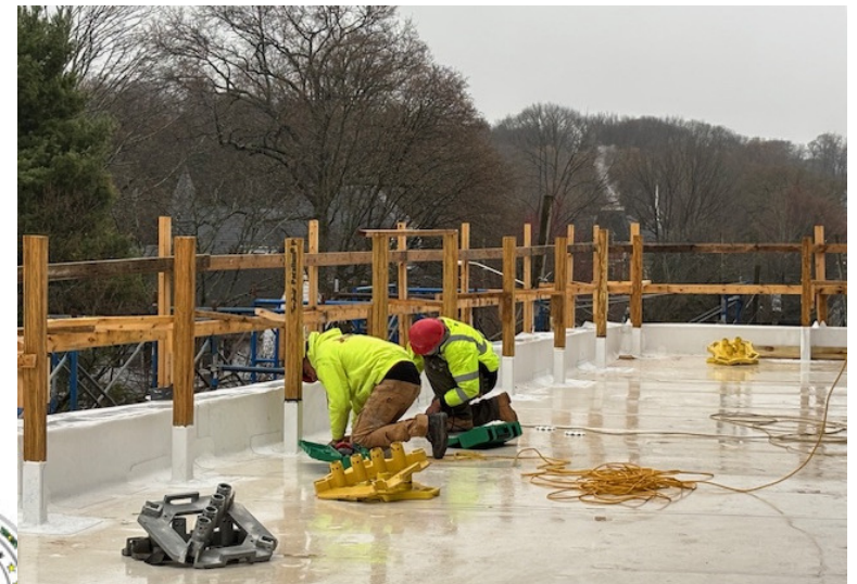
Work on Roof Deck
