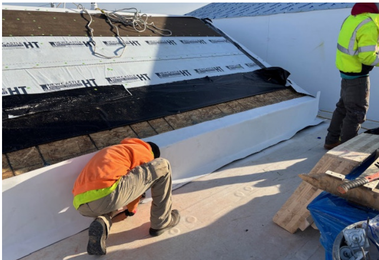
Roof Flashing Ongoing
