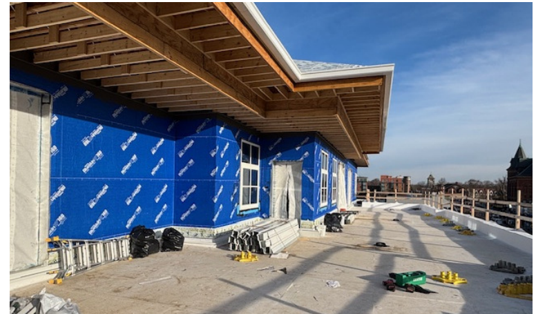
View of Building from Roof Deck
