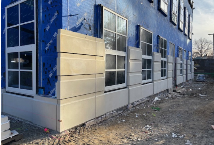
Precast Installation Ongoing – South Elevation Shown
