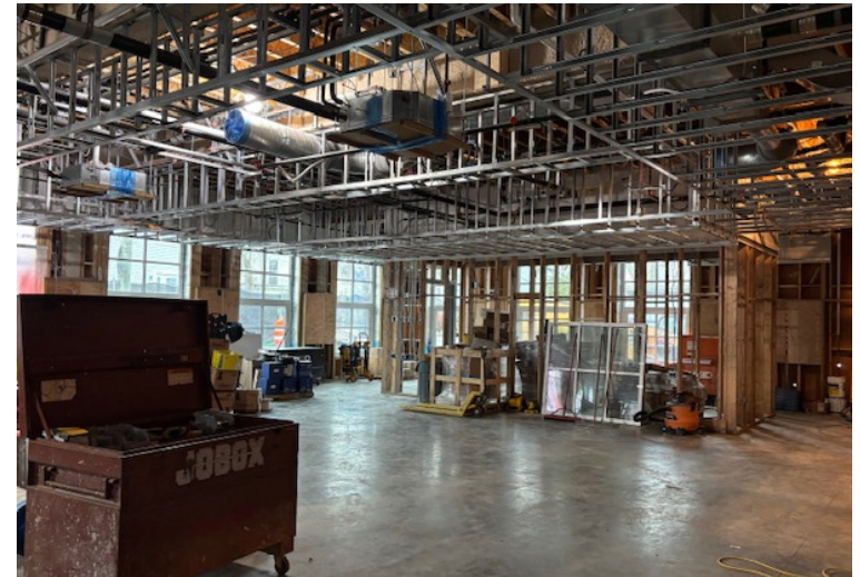
Metal Soffit Ceiling Framing in Multi- Purpose Room
