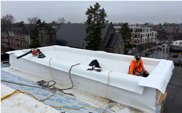
Installing Roofing at North Stair Tower
