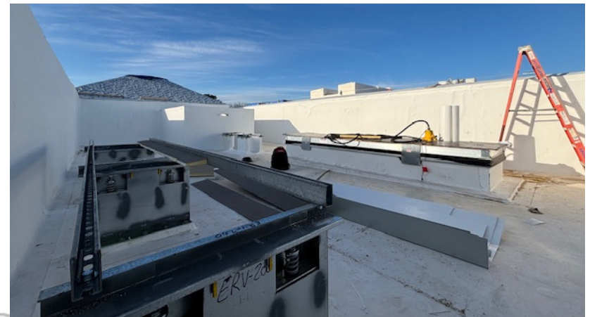
Roofing complete awaiting rooftop equipment
