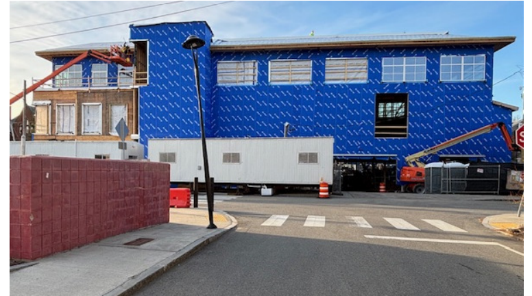
Exterior View from North
