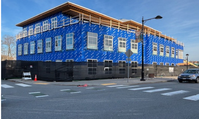
Exterior View from Southeast
