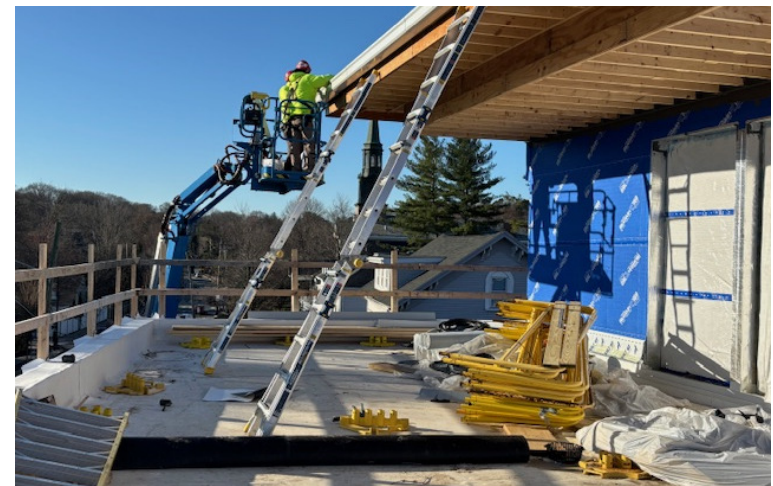
Gutter Installation Ongoing at Sloped Roofs
