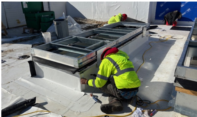
Installing Mechanical Equipment Curb
