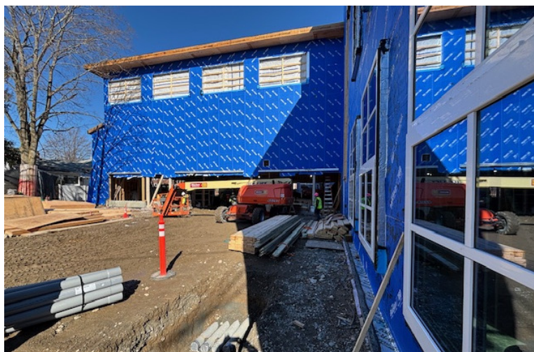
Exterior View of Gym from Southeast
