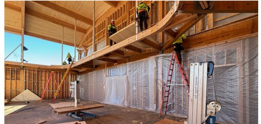
Walking Track Deck Installation
