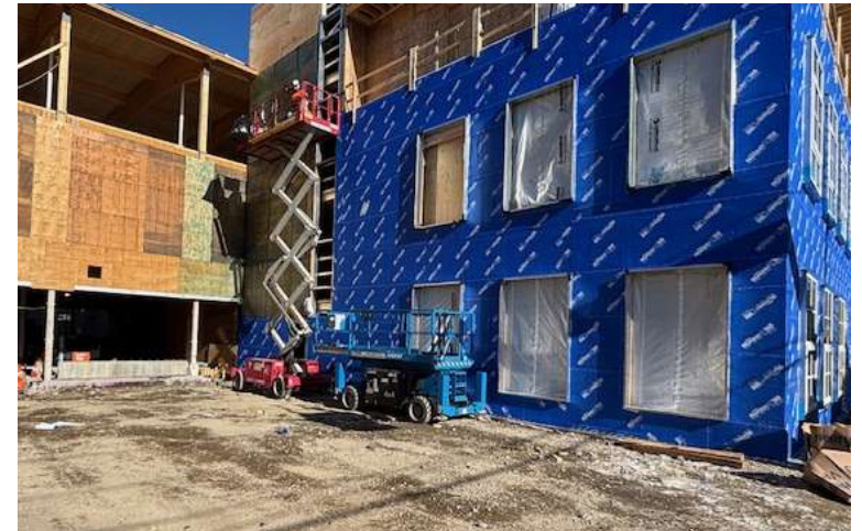
Air-Vapor Barrier installed on West wall
