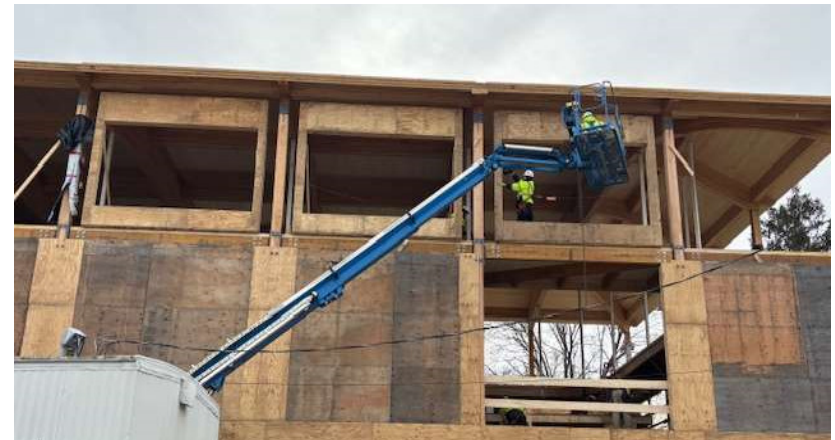
Gym Wall Panel Erection on North Elevation
