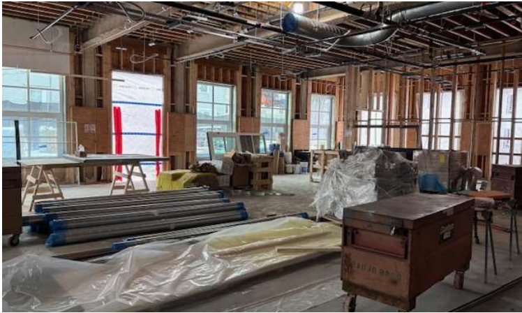
Multi-Purpose Room Rough-in
