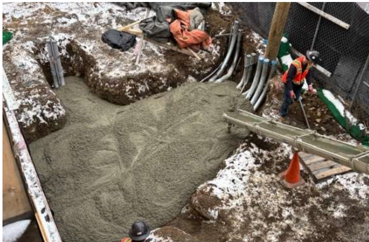
Generator Ductbank
