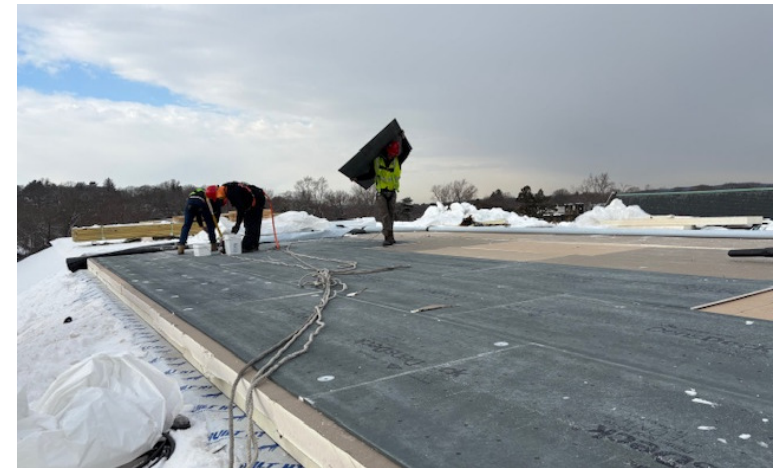
Gym Roof Underlayment Installation
