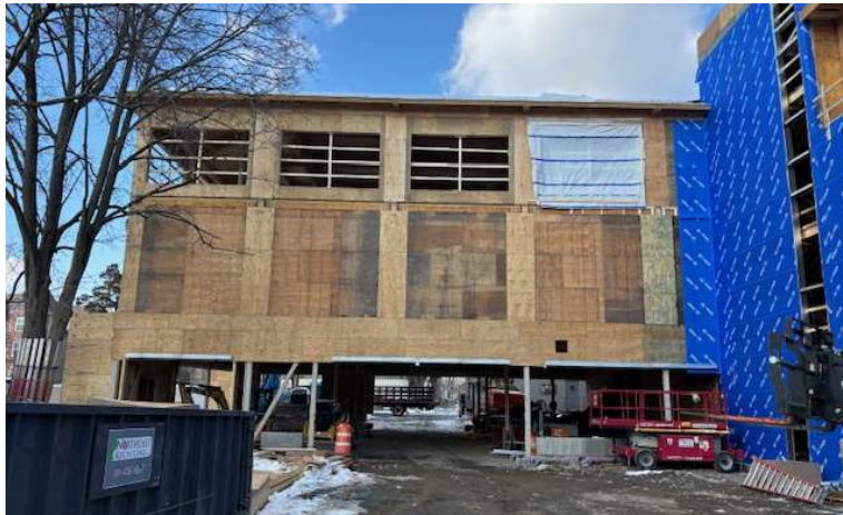
Gym wall panels complete on South wall
