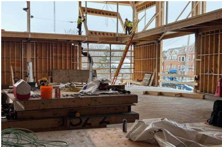
Gym Wall Panel Erection
