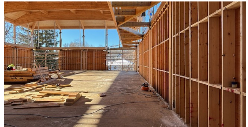
Walking Track Deck Framing
