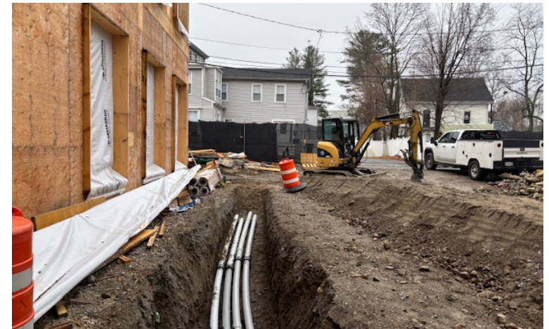
Electrical Service (Secondary) in process
