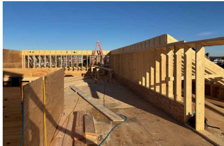
Roof Framing at High Roof
