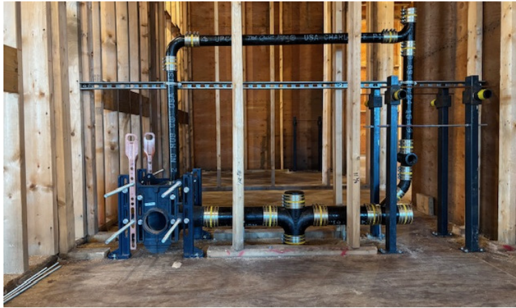
Rough Plumbing under way
