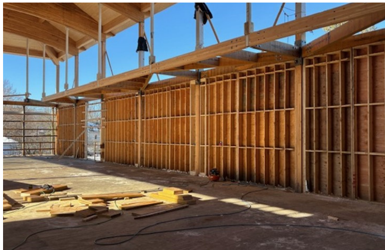
Walking Track Edge Beam and Framing
