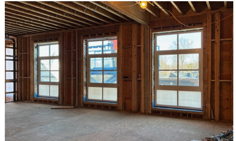
Windows Installed at Second Flr. Art Room
