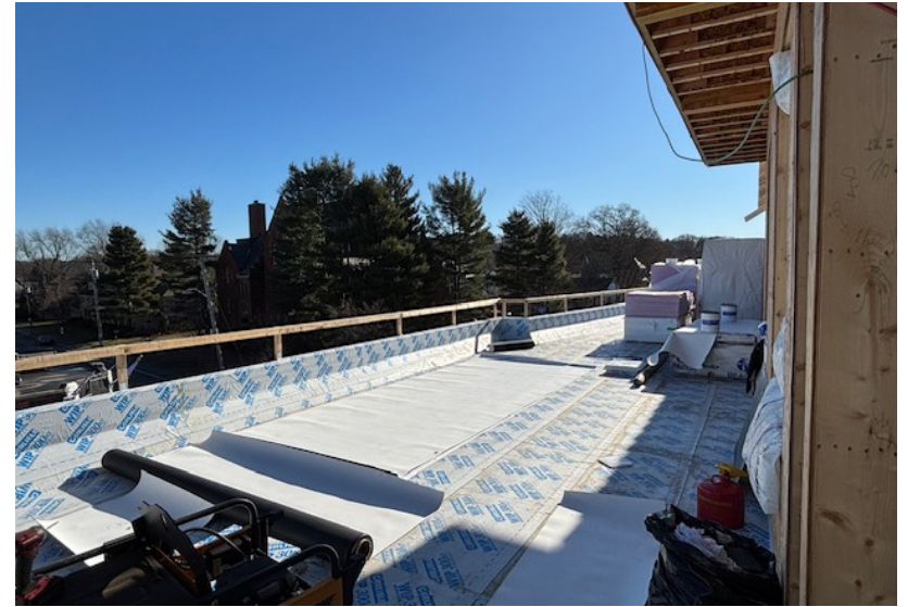
Roof membrane in process at Deck
